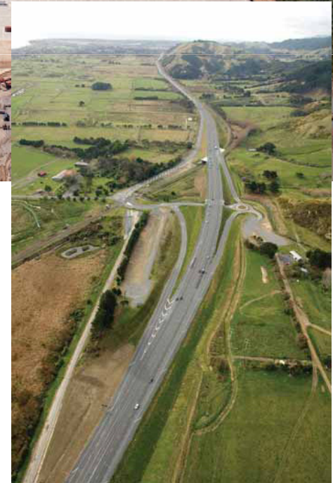
SH1 MacKay's Crossing
