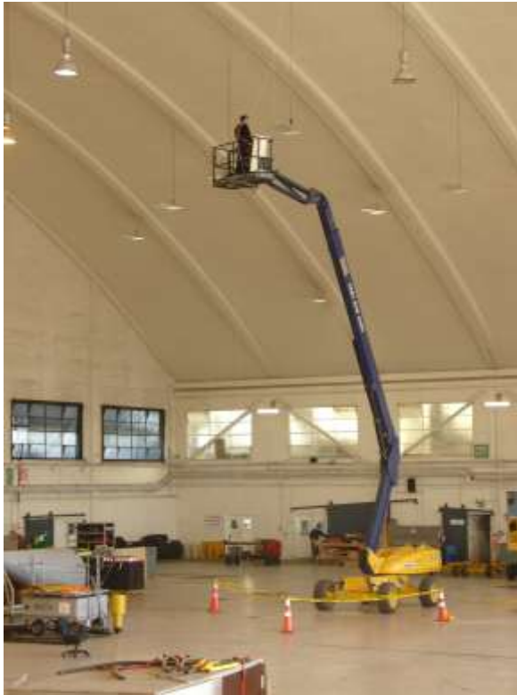
5 Sqn Hangar Lighting Change Project
