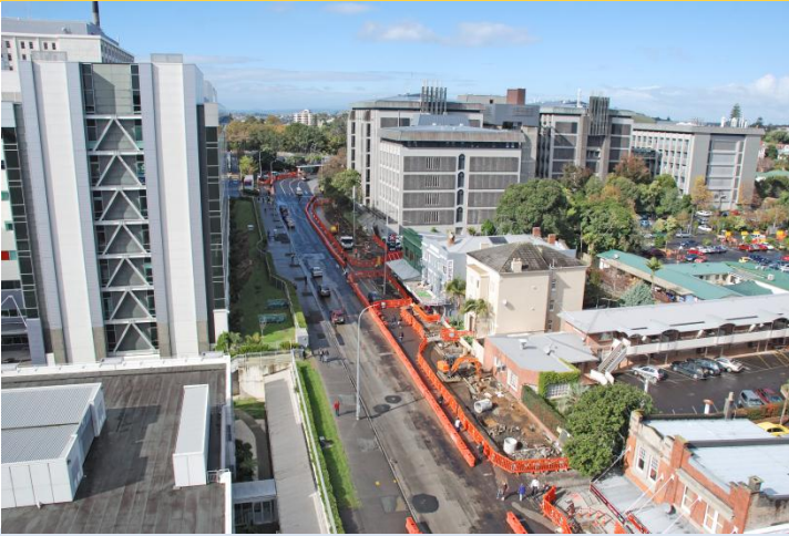
The Central Connector Project in progress.
