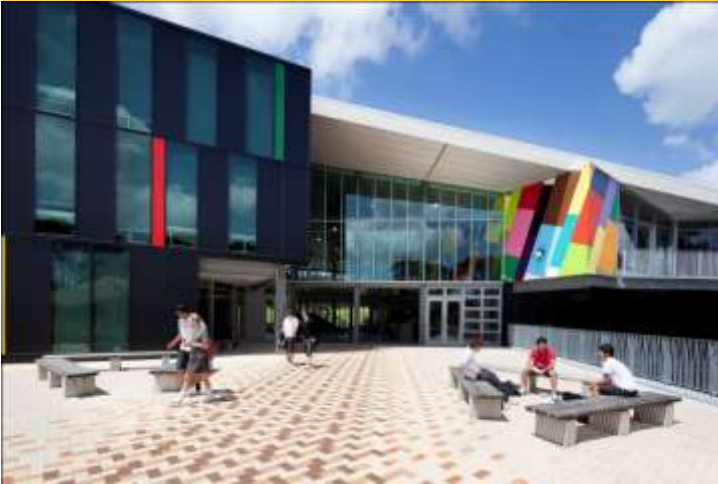
A view of the new Albany Senior High School
