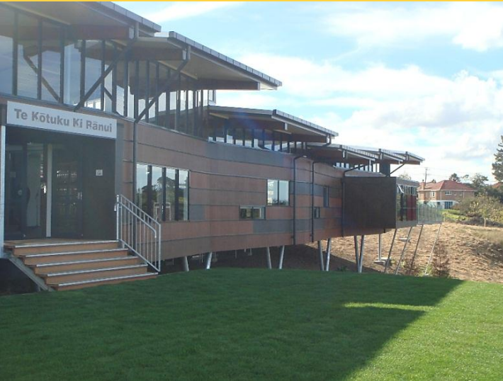
A side profile of the school and its entrance
