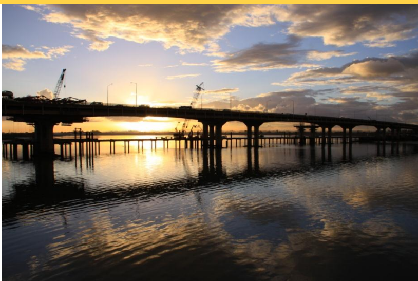
Early in the project: the existing bridge in the foreground
