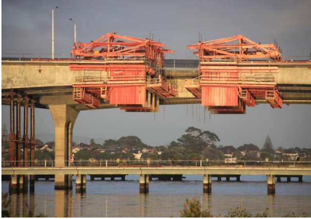
The north and south sections are prepared to be joined
