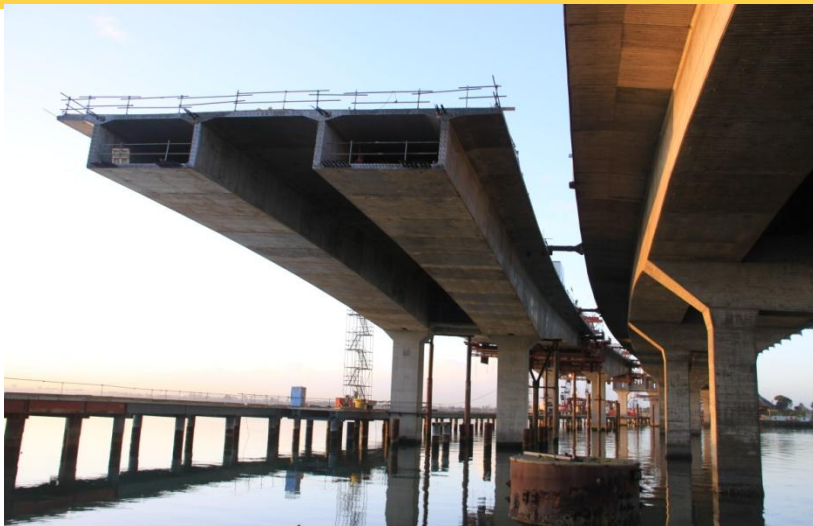
The new structure adjacent to the existing bridge
