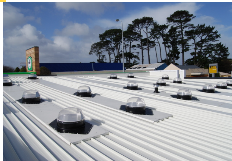
The roof showing the Sola Tube Skylights which provide natural light to the interior
