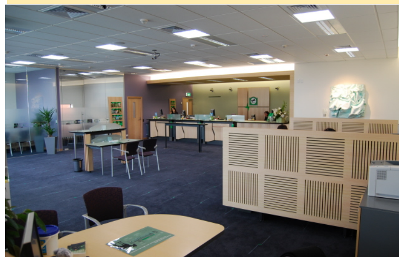
The completed branch Interior showing daylight diffuses and adjacent flourescent lights on adjustable light sensors
