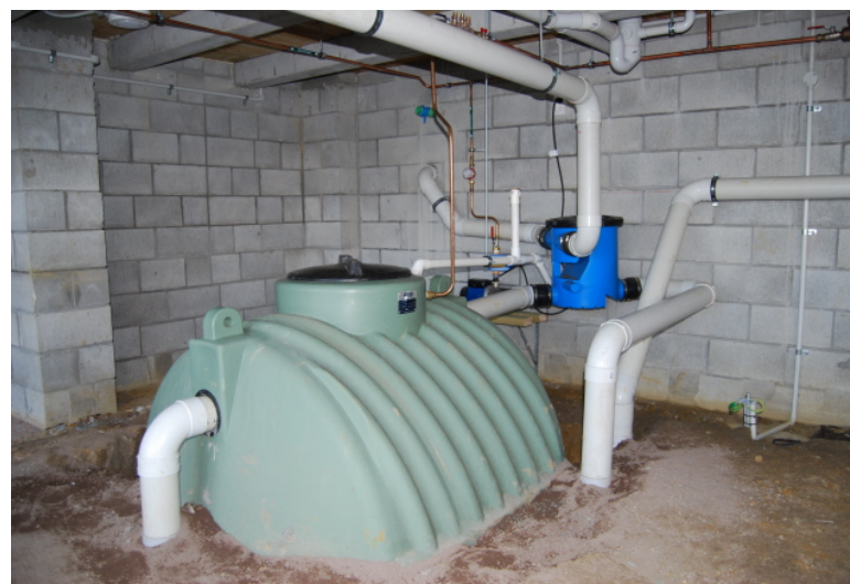
The rainwater harvesting tank for the toilets and cleaner's sink
