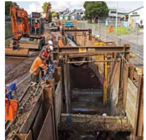
▲ The NEC-procured first stage of the Hunua 4 water main is being constructed predominately in open-cut methods
