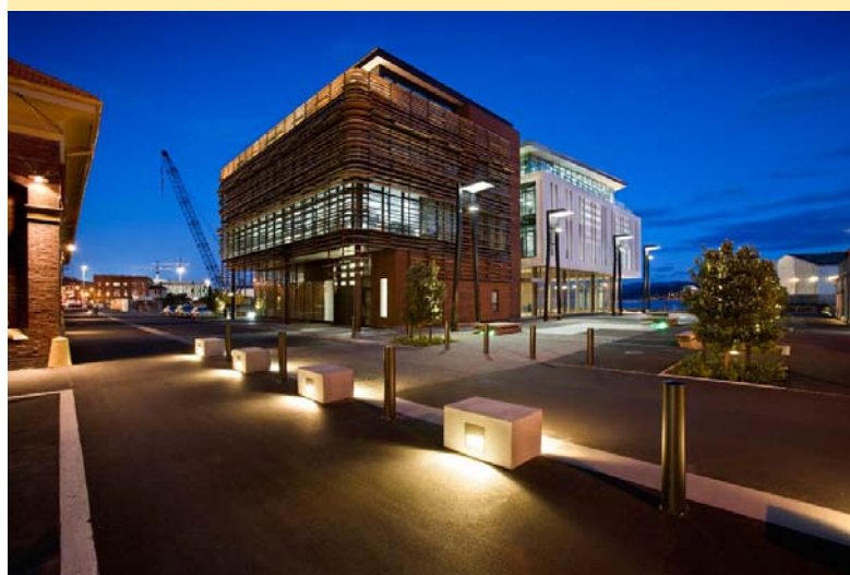
Meridian Building South West corner, looking along the lane from Wharf Plaza. Photograph provided by Simon Devitt, Photographer.
