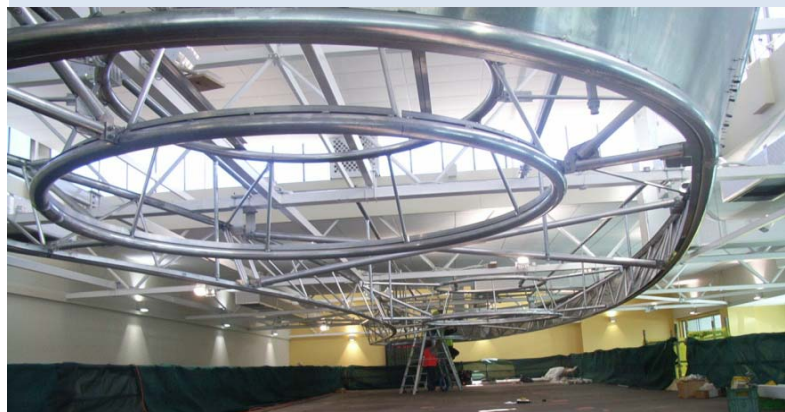
Erecting the barrisol frame and fit out installations had to be done overnight as the airport operates 24/7
