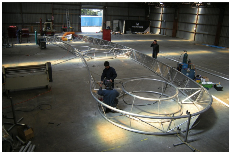
The ceiling barrisol framing presented a significant engineering challenge
