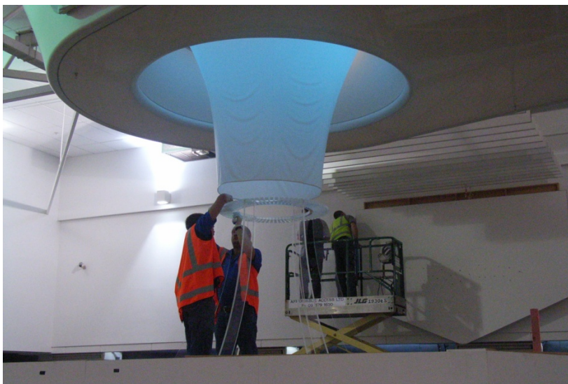
The barrisol material had to be specially flown in from France
