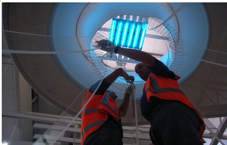
Installing the purpose designed kiosk cluster acrylic
