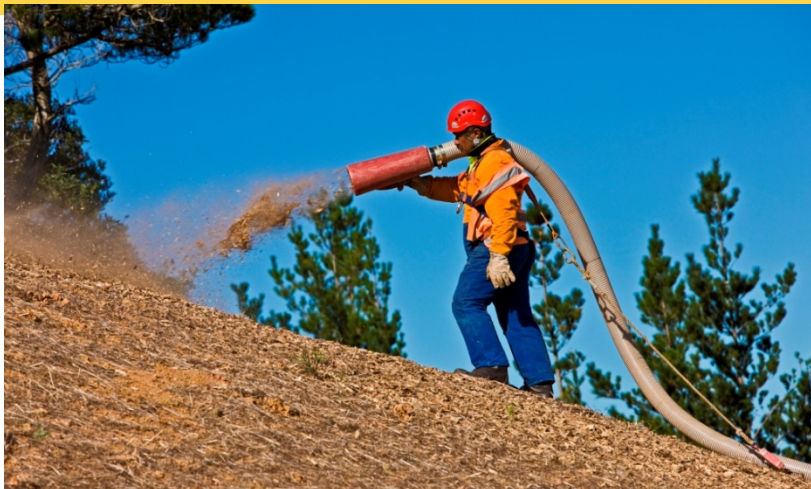
Mulching of slopes for planting
