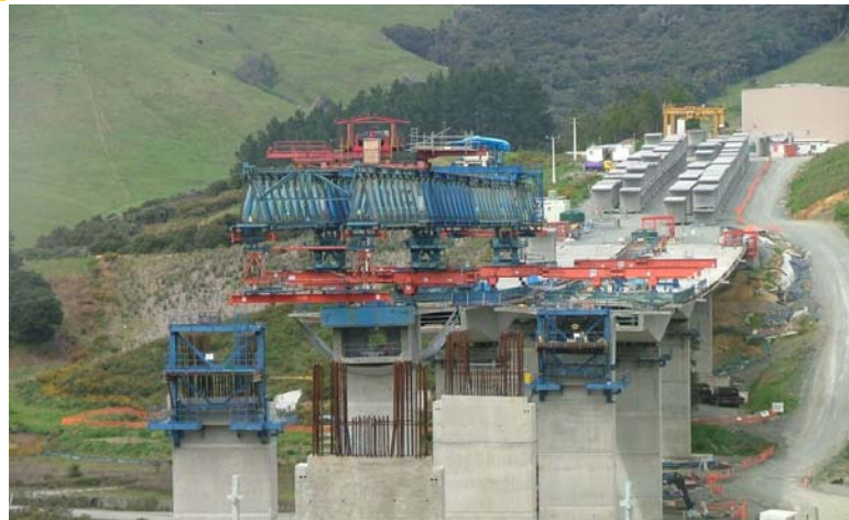
Construction of the Waiwera Viaducts
