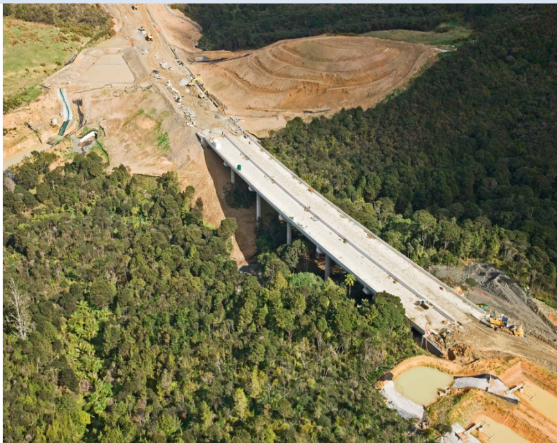
Nukumea Eco-viaduct under construction
