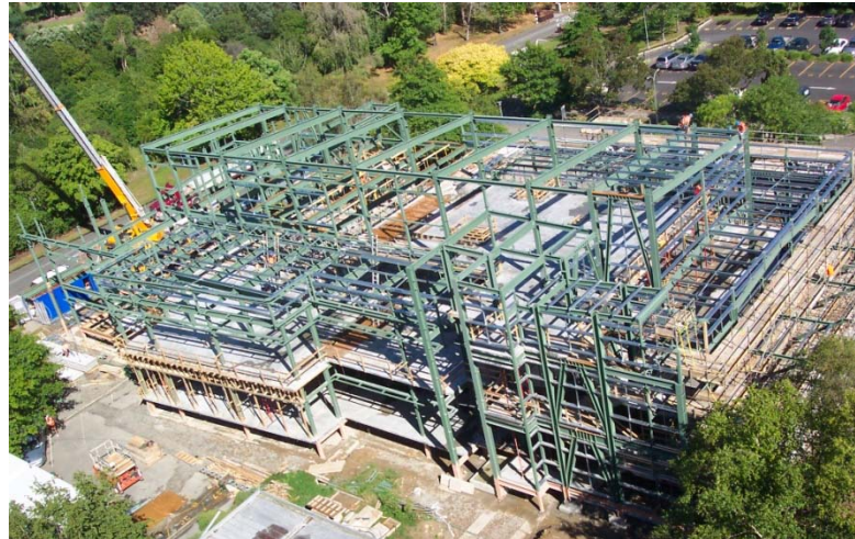
The Project at 25 th January 2006
