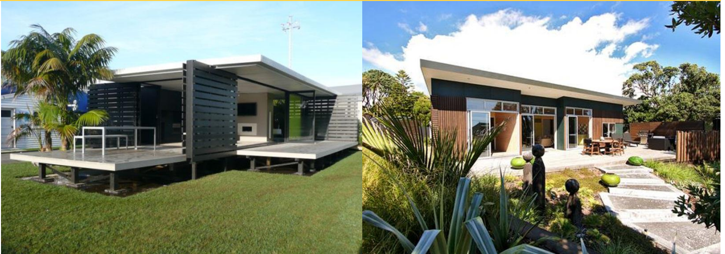
NZ Prefabrication: iPad (left) and K-Bach (right)
