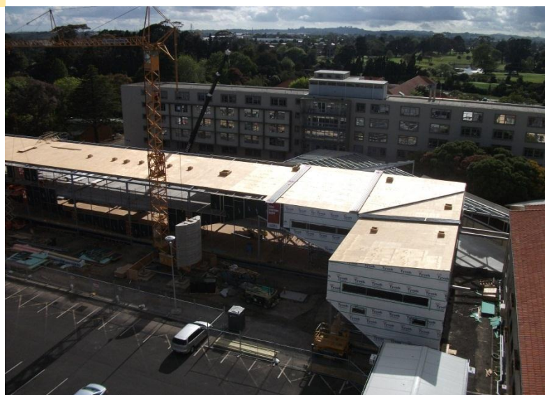
Prefab in-use: Pathfinder 26 Middlemore Hospital
