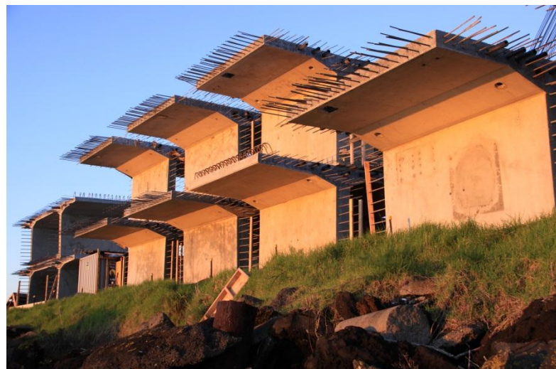
Prefab in-use: Pathfinder 15 Manukau Harbour Crossing Alliance
