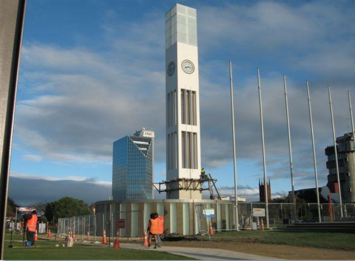
The refurbished Hopwood clock tower approaching completion.
