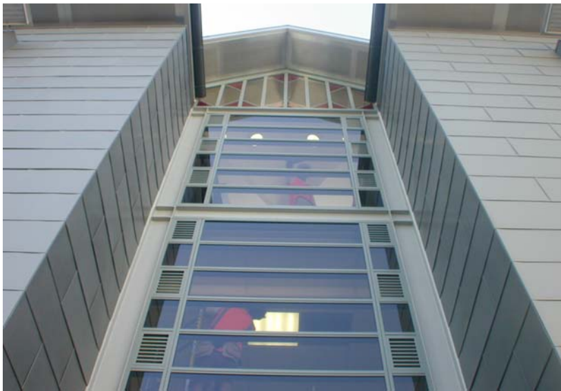
Detail of the Rutland Street facade showing the cladding.
