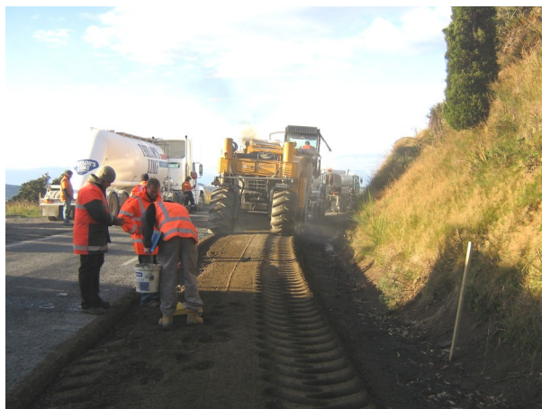
Cement stabilisation of a highway shoulder.
